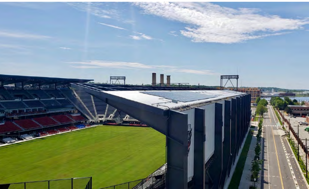
The rooftop and canopy PV system at Audi Field will generate over 787,000 kilowatt hours of renewable energy and cut CO2 emissions by 556 metric tons each year
