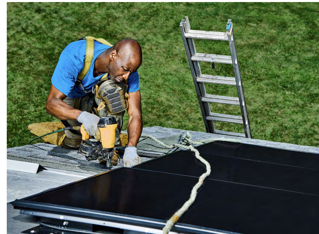
A technician installs an integrated solar roof. Aesthetics and speed of installation are key issues for GAF Energy.
